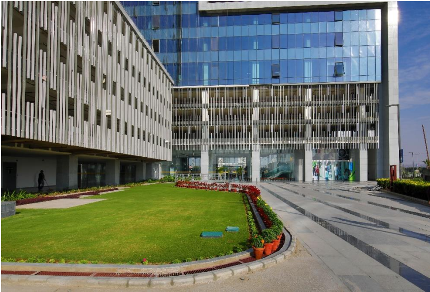
View of Drop-off Area
