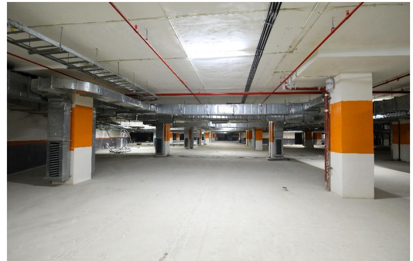
Actual Image of Basement Area
