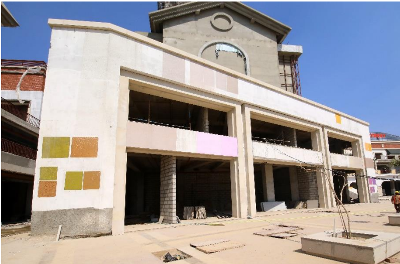
Finishing Work of Shops in Progress
